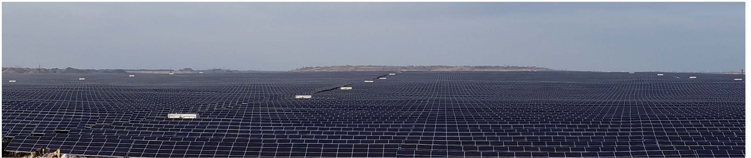
Ukraine 200MW PV Plant
